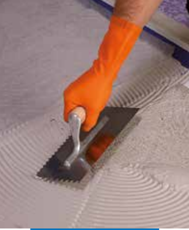
Applying a first layer of Monolastic welded with Mapetex Sel on a new screed
