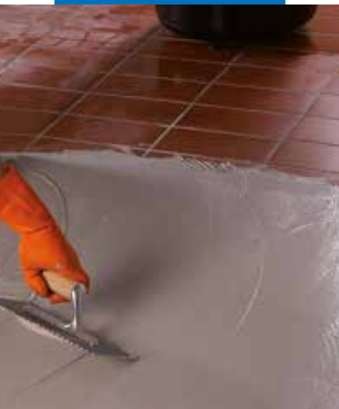
Applying a second layer of Monolastic on Mapebet 150
